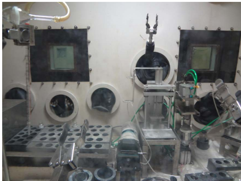
Figure 10: Liquid transfer machine and other accessories inside the STB.
